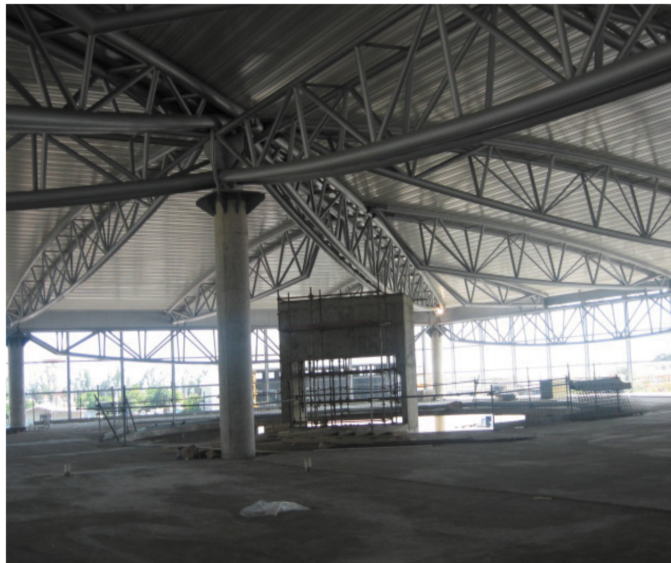
MAIN ROOF SUPPORT TRUSSES
