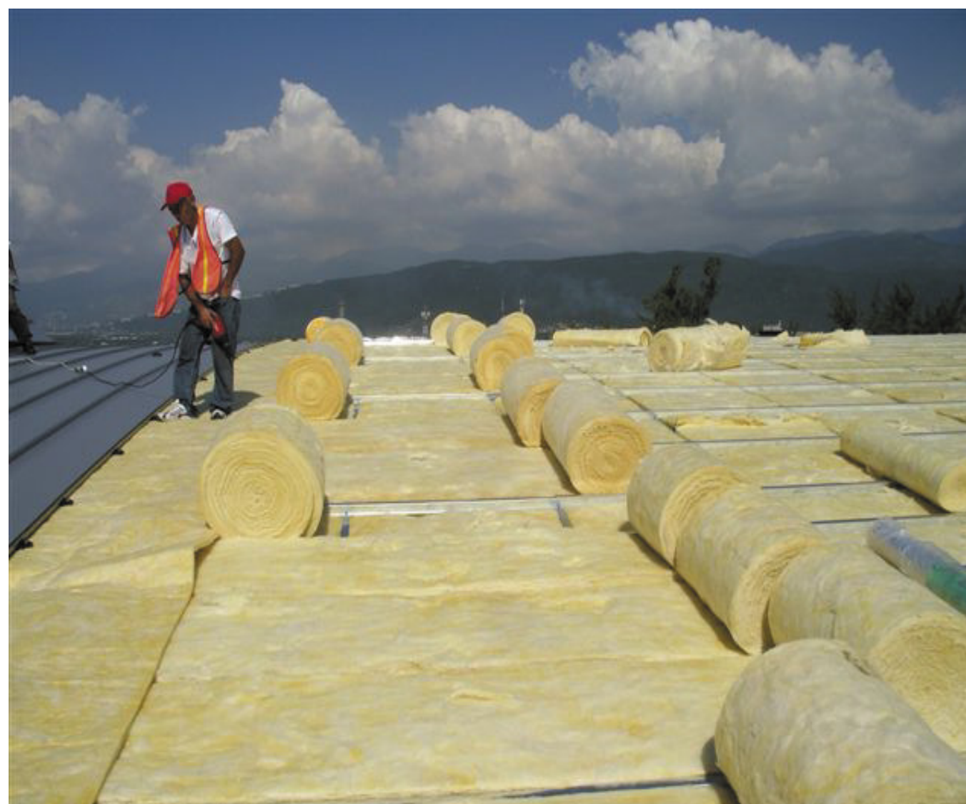
INSTALLATION OF ROOF INSULATION
