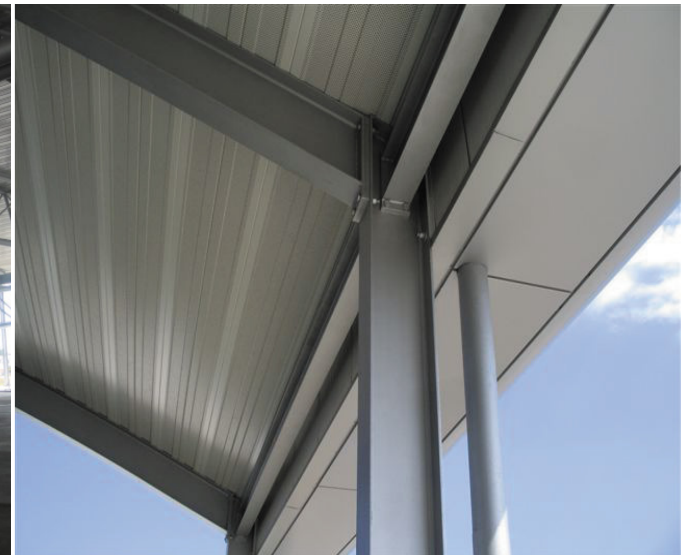
ROOF STEELWORK SUPPORT TO STEEL ROOF SHEETING
