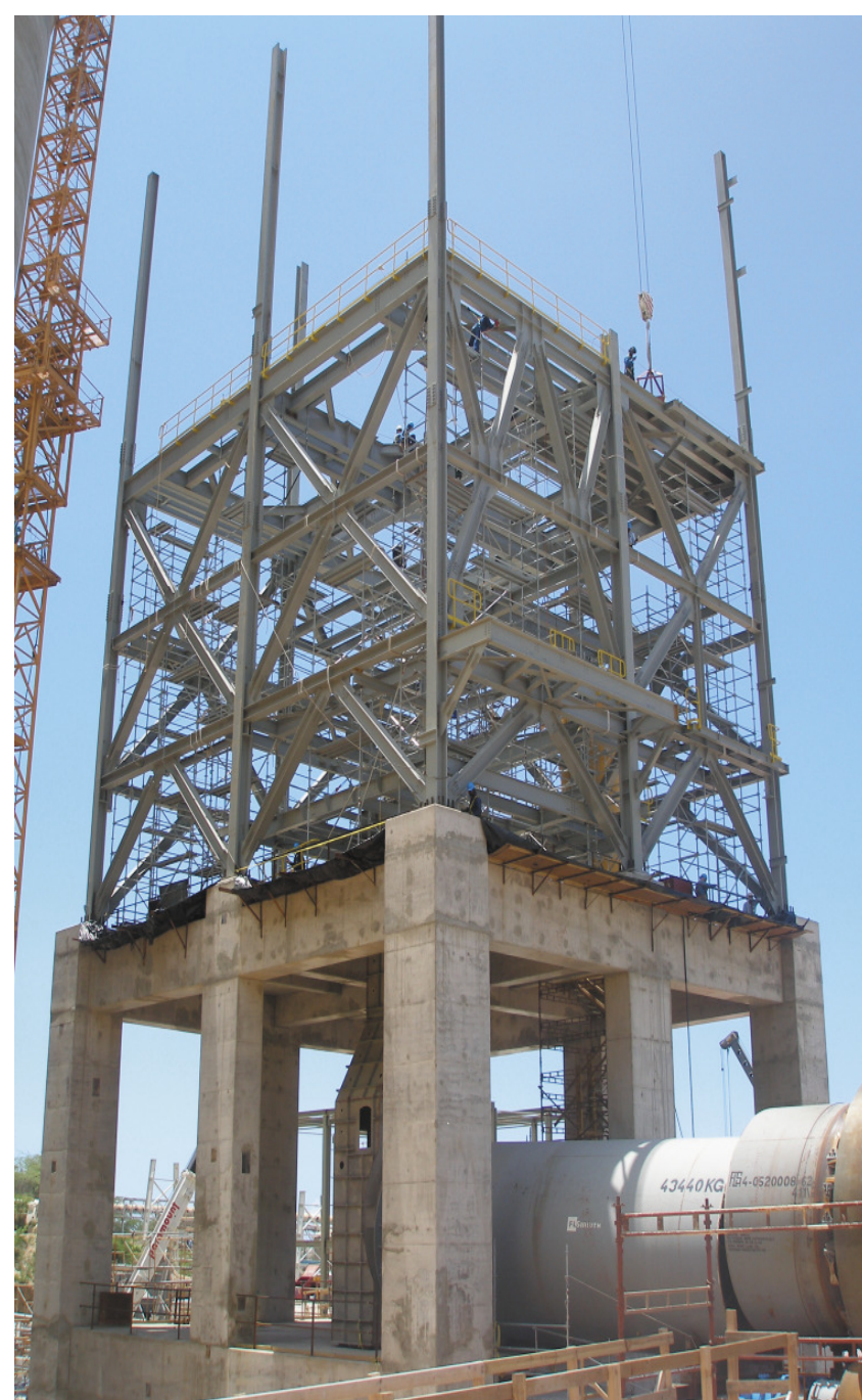
ERECTION OF STRUCTURAL STEELWORK ON RC FRAME
