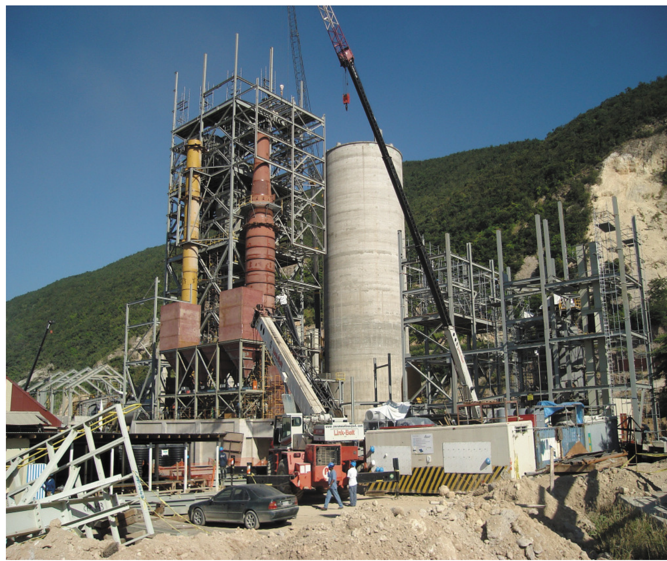
COMPLETED CONCRETE KILN WITH STRUCTURAL STEELWORK FRAMING ADJACENT
