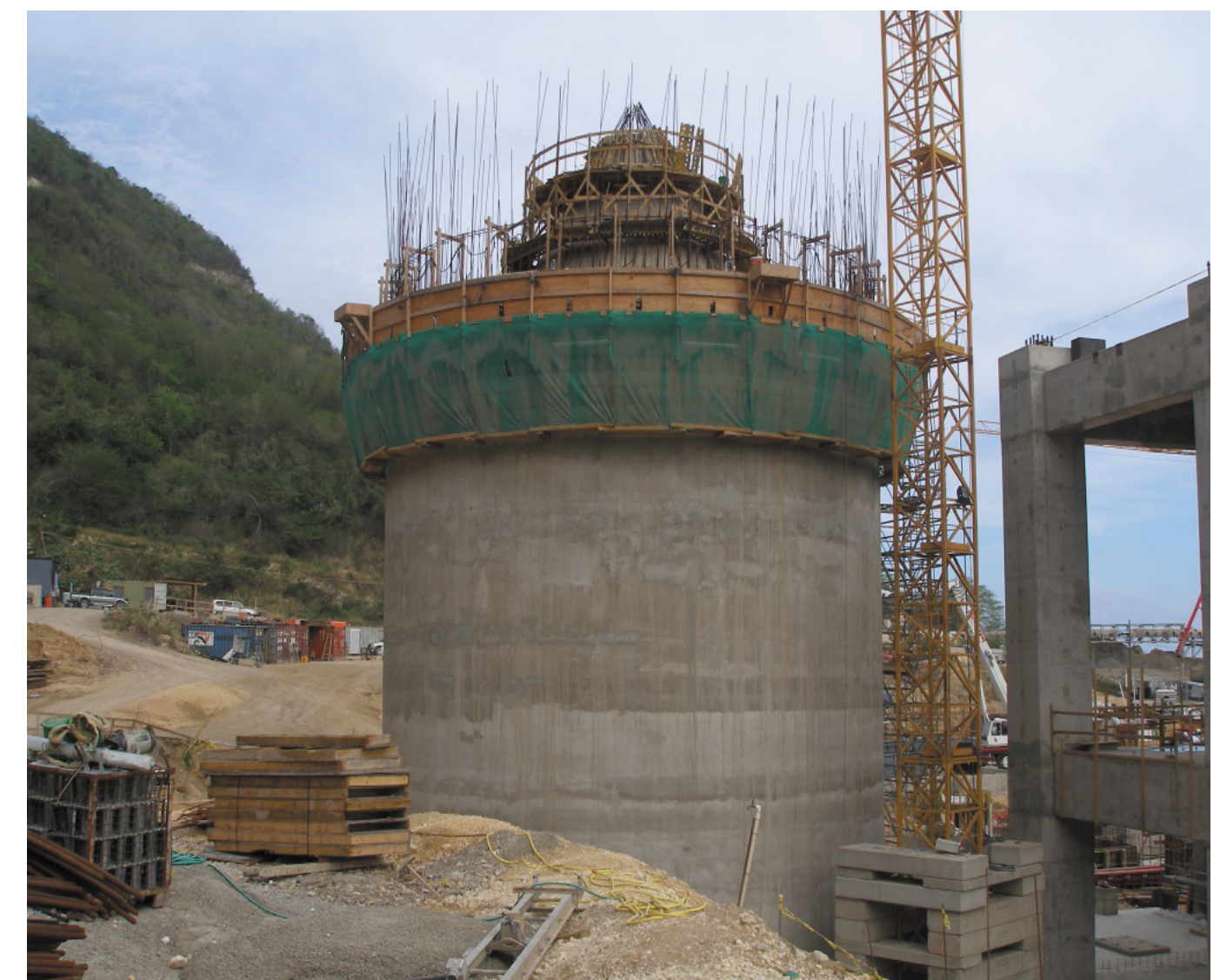
FORMWORK & CONCRETE PLACING TO KILN
